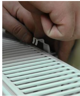
Slide the top clamp down tightly onto the radiator. The fingers of the clamp should fit between grills.
