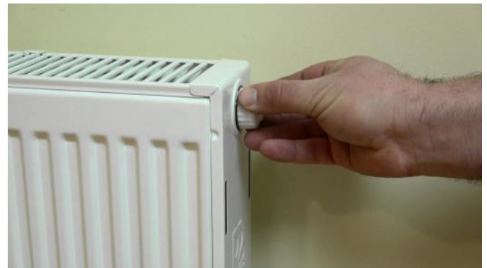
Turn the knob onto the Thermostatic Valve by turning clockwise. Initially only turn the knob 1/2 to 1 turn.
