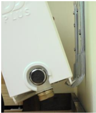
Set the bottom rear of the radiator in the groove at the bottom or each bracket and tilt the radiator till vertical
