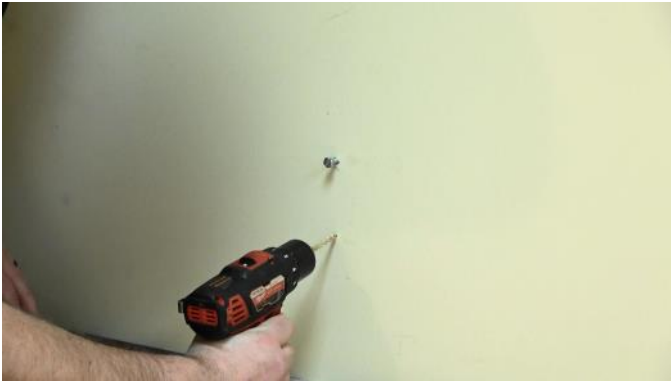
Remove the mounting bracket and drill an appropriate pilot hole for the lower mounting bracket bolt.
