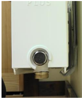
Set the bottom rear of the radiator in the groove at the bottom or each bracket and tilt the radiator till vertical
