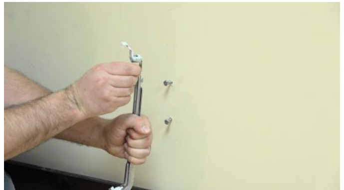
Pull the white tab forward and slide the top clamp upward to raise the clamp to its highest point.
