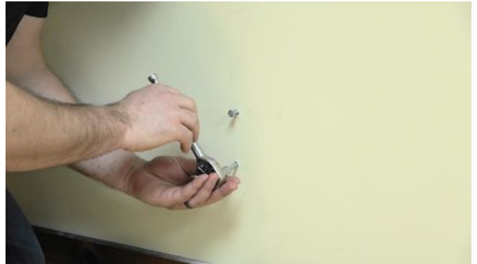
Insert the lower mounting bolt and tighten with a wrench till bolt head is about 3/4" from wall.
