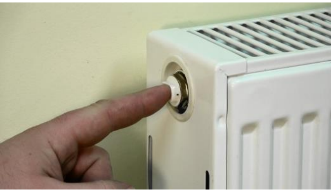
Locate the small vent hole in the side of the white plastic portion of the air vent.
