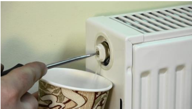
Hold a cup or other suitable container under the vent. Insert a flat screwdriver into the chrome slotted nut on the vent.
