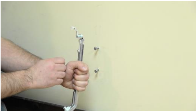
Grip the bracket in one hand. With the other hand grip the white plastic tab at the top of the bracket.
