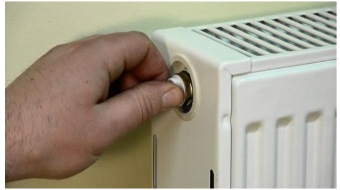
Rotate the white portion of the air vent until the small vent hole points down.
