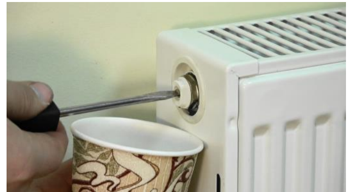
Once all air escapes and a steady stream of water flows from the vent, rotate clockwise until the flow of water stops and the vent is tight.
