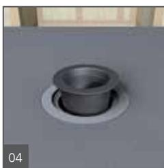
04 Drop the drain body firmly into the sealant.
