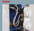
Screw terminal where a wire pushed back into the work
