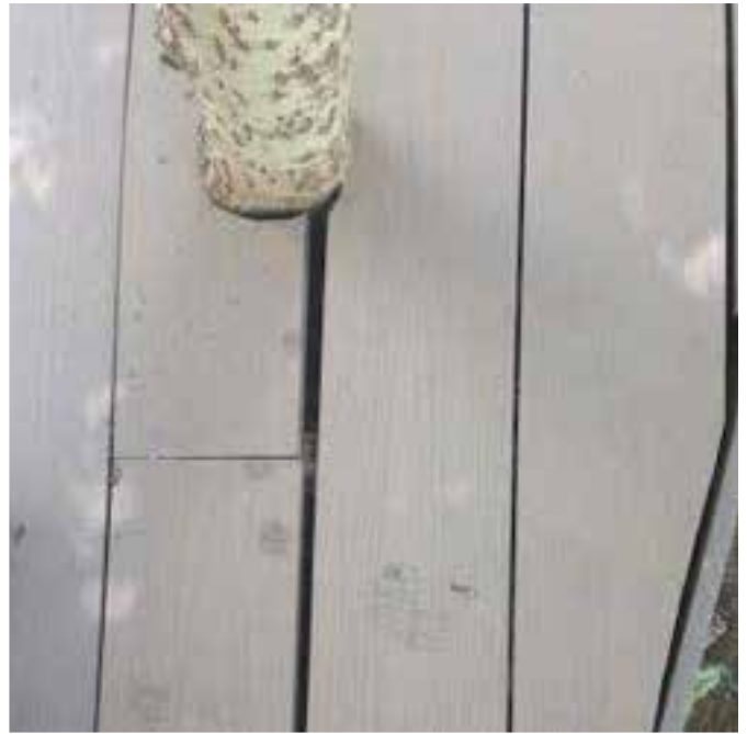
Tree has grown more than allowable cut out. Leave sufficient gaps for the plants and trees to grow.
