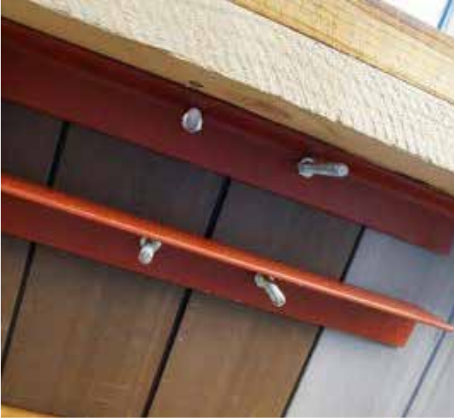
The railing post is only supported by the decking. Proper blocking should be installed to support the railing post.
