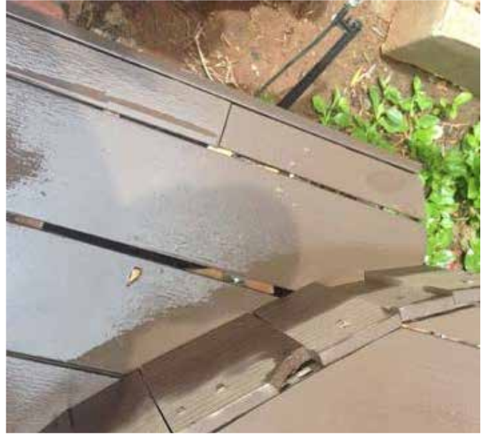
Improper fascia installation.
