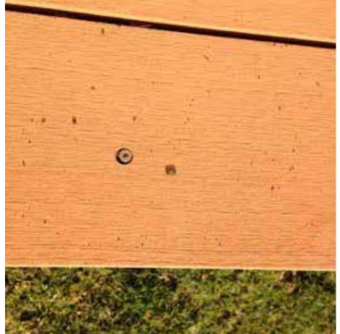
Counter sink is too deep and too big for the size of the screw.
