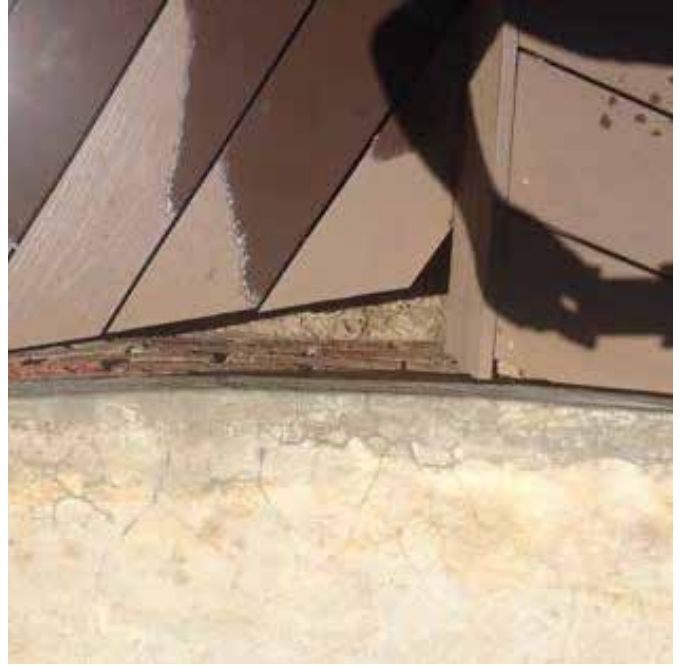
Poorly planned installation.
