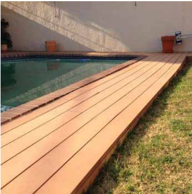
Sloping away, either the earth has dropped or the frame has dropped. There is also insufficient drainage.
