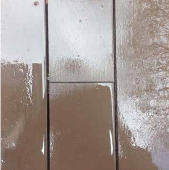
No double joist and no double clip at the butt joint.
