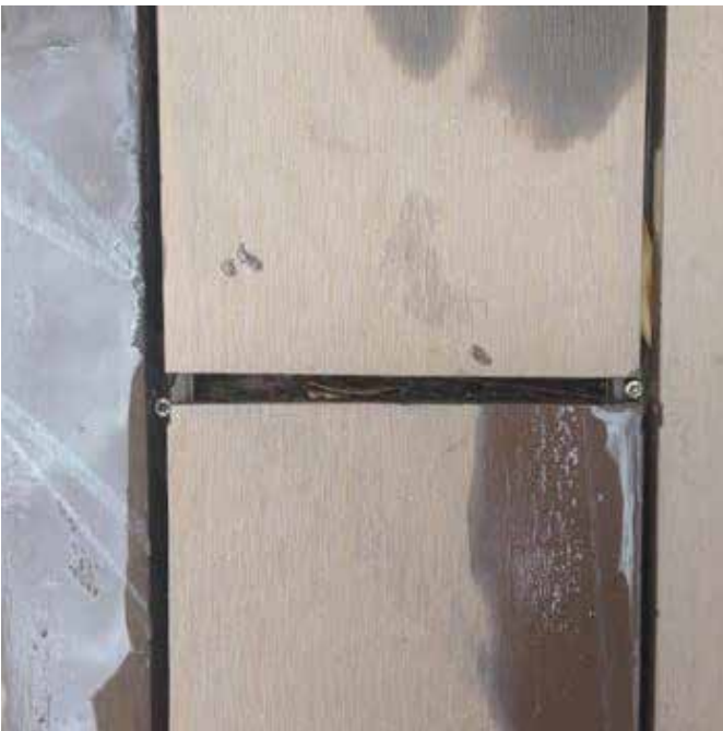
No double joist and no double clip.
