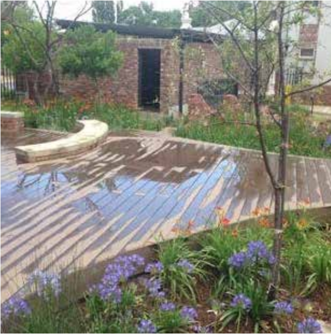
Deck is not sloping away, this deck is sloping to the center.
