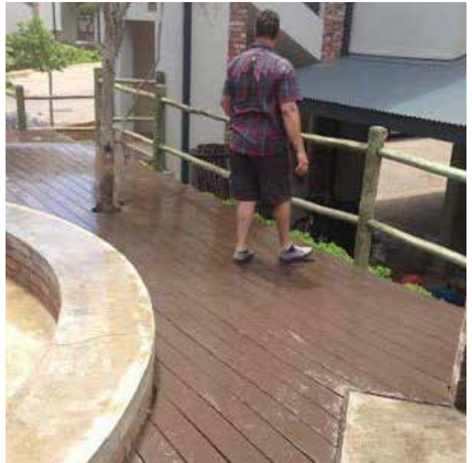
Deck sloping away, frame is giving in.
