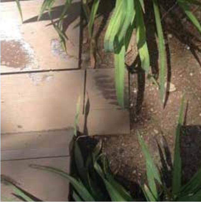
Unfinished cutting left. Nobody checked the deck after completion.
