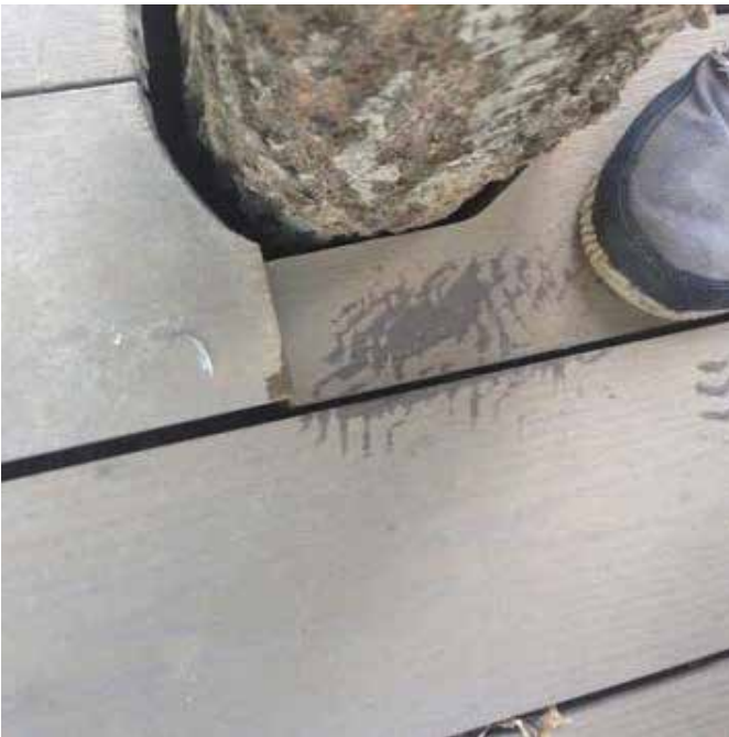
Improper blocking. No support under the decking.
