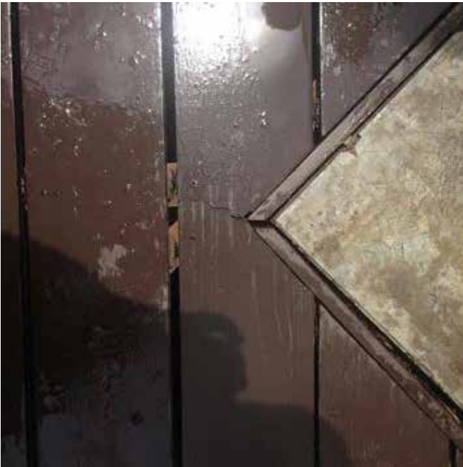
Cracked deck board installed. Cracked deck board installed.
