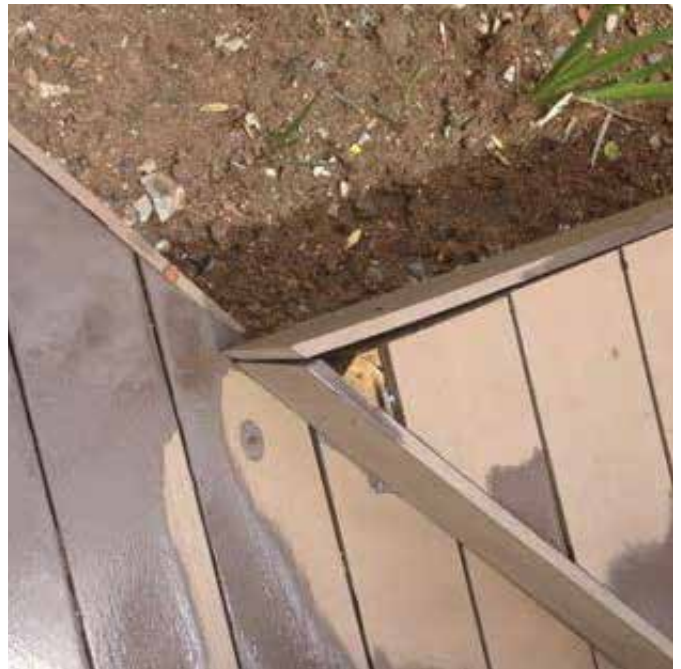
Missing piece of decking. Fascia not cut correctly.
