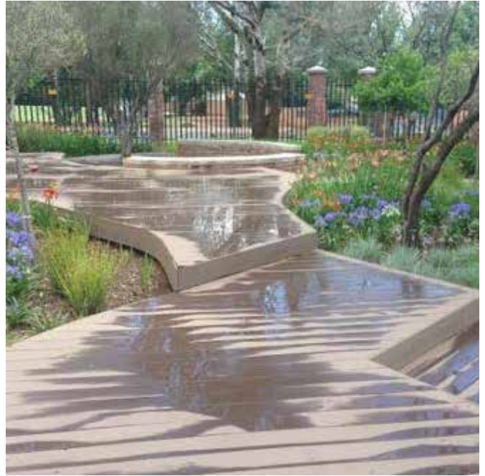
Deck is not sloping correctly. Water is collecting in the center of the boards.
