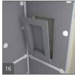
2 Fasteners on each side of the niche are set to create a flush transition to the wall panels. Another 1/2" (12.7 mm) bead of wedi Joint Sealant is spread over fasteners and seams.
