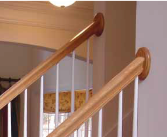
ATTACHING RAIL WITH A ROSETTE
