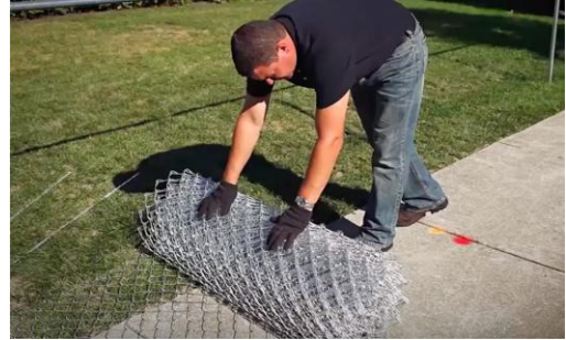
Roll the mesh out along the fence line.
