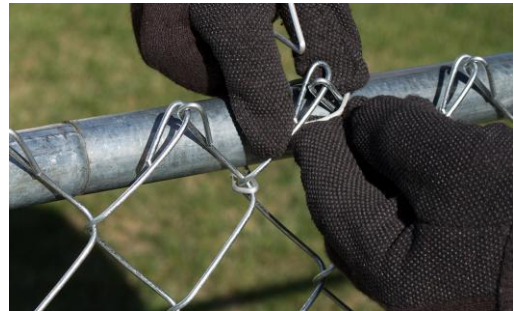
Fasten the bar to one side rail.
