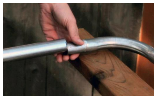
Slide the tubing together, add bands.
