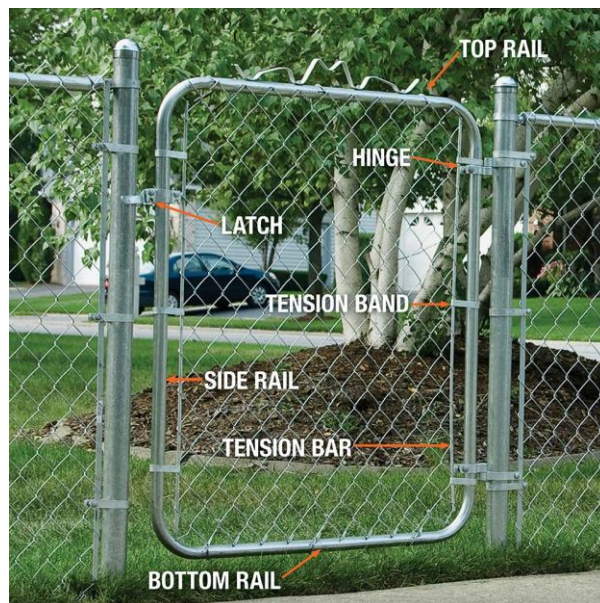
The parts of a chain link gate.
