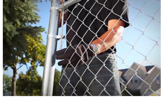
Set a tension bar before releasing tension.
