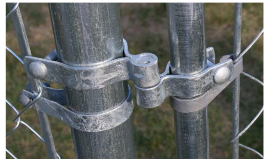
Top pin down, bottom pin up.
