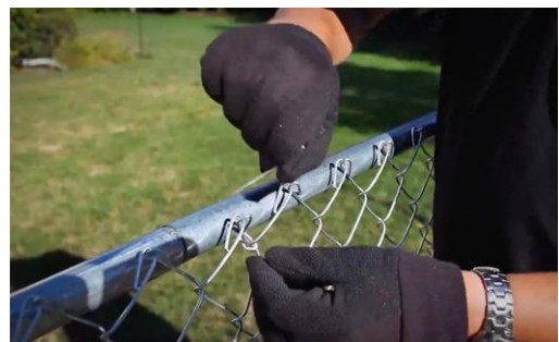
Tie wires hold the fabric to the rail.
