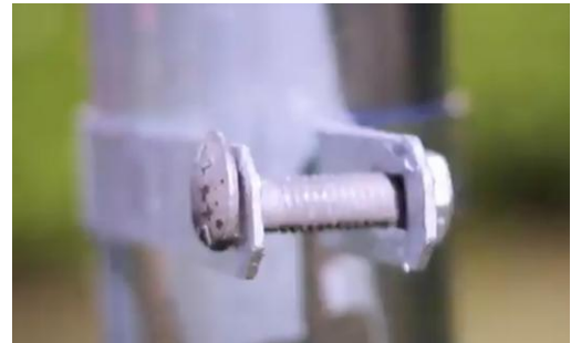
Mount straps flat side up, evenly spaced.
