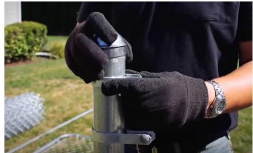
Feed the top rail through the looped caps.
