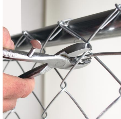
Tie the top and bottom for a clean edge.
