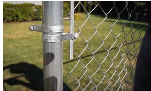
Bolt the bar into the tension bands.
