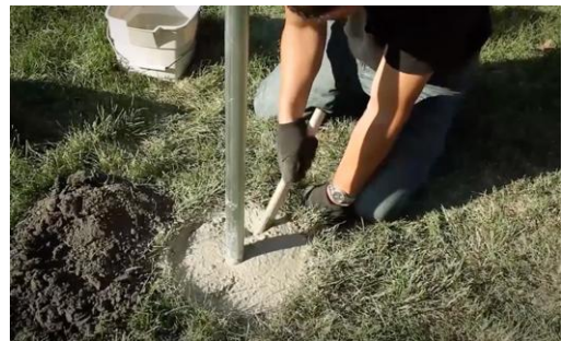
Set terminal posts plumb in concrete.
