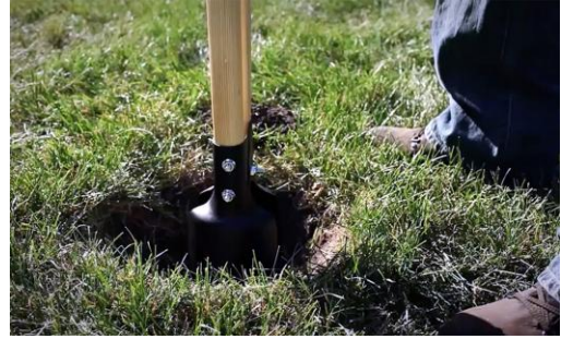
Dig each hole to the right width and depth.
