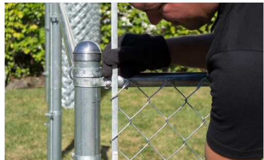
Pull the mesh taut, then slip the bar in.
