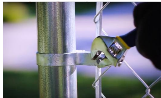
Draw the bar in and tighten the bolts.
