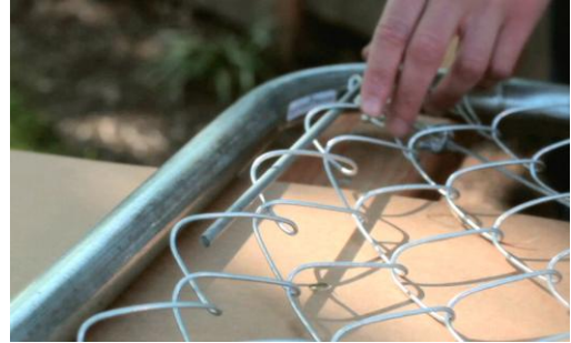
Thread the bar through the full width.
