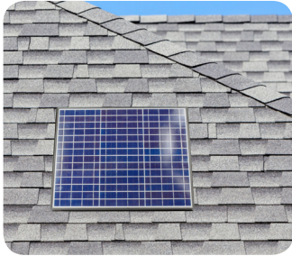
Surface Mount on Shingle Roof
