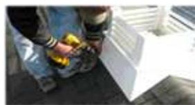
**Step 9:** Position cupola on center of roof and fasten with 3" white headed screws. **Note: if you want to utilize venting, cut a hole (app. 8" square) in the roof prior to fastening cupola. Attach screen mesh over hole to keep bugs out.)**
