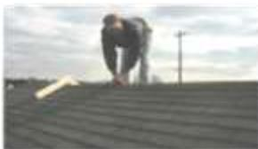
**Step 2:** Measure overall length of roof; find center and mark.
