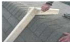
**Step 3:** Lay your boards over the peak of the roof, making sure each board is fully against the surface. Mark boards with pencil to confirm angle position. Mark front & back of roof (not all roofs are symmetrical.)
