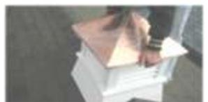
**Step 10:** Place cupola roof on top of base. **Note: Remove shrink wrap from copper after Step 9 is done, to protect copper from oils on skin.**
