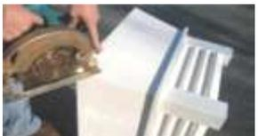
**Step 8:** Cut out roof profile by starting at corners of cupola base and cutting to the center. Repeat steps 4 - 6 on the opposite side of your cupola base. (If your roof is not symmetrical, make sure that your lines / cuts match the angles needed for the front and back roofs.)
