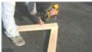
**Step 1:** Use 2 pieces of wood each ~ 24 in. long (2x4s are ideal). Fasten together with one screw, just loose enough that boards can still pivot with pressure.
