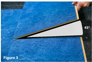
5. Slide it gently to the left. Lower it into the groove of the first piece and press it into place. You should hear a "clicking" sound when it locks into place.
