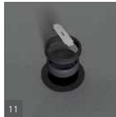
Tighten (squeeze) the rubber caulking gasket firmly with the caulking nut (use a flat headed screwdriver) and finally insert the plastic frame and strainer on top (without adhesive). The frame and strainer will be held in a grout joint only once tiling commences. Do not tighten the gasket prior to 60 minutes after the threaded drain part was sealed into the shower base.
