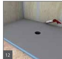
Set up a continuous 1/2" (12.7 mm) bead of wedi Joint Sealant along the pans channel on the outer perimeter and only in areas where you can immediately install a wedi Building Panel into the fresh sealant.
