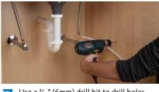
Use a ½2" (6mm) drill bit to drill holes. Carefully tap the plastic anchors into the drilled hole with a hammer. Mount unit to the wall with the screws. Pull the protective plastic strip from the battery compartment. The red LED should flash and beep five (5) times to indicate that the battery is installed correctly.
