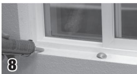
**8** Apply 1-inch balls of polyurethane construction adhesive 3 to 6 inches from each end and 12 inches on center of the sill area.
