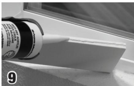
**9** Apply a bead of caulk to the back edge of the sill.
