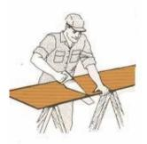
If measured floor-to-ceiling height is 8' or less, subtract ½" from this measurement to allow ¼" expansion clearance on top and bottom. Transfer these measurements to panels for cutting. If using a handsaw or table saw, mark and cut the panels face up. If using a portable circular saw or sabre saw, mark and cut panels face down. Cutouts for door and window sections, electrical switches and outlets or heat registers require careful measurements.
