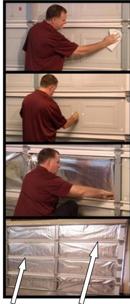
**For improved thermal performance, add 3/4” air space between Reflective Air and door. This can be done by attaching to door framing rather than to the door panel**
