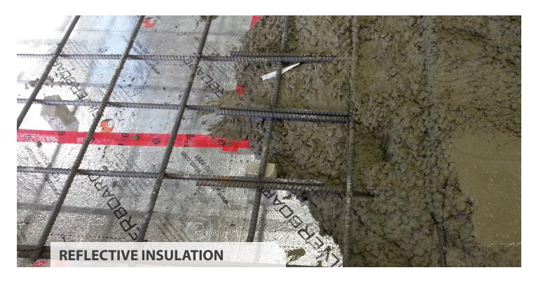
SilveRboard is a non-structural, rigid insulation board made from Expanded Polystyrene (EPS) with a layer of reflective metalized polypropylene film lamination on both sides.
