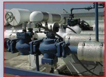
Maintaining ammonia refrigeration piping
