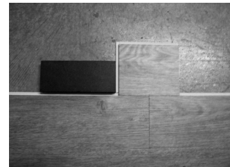
Fig. 7 – Tap side of plank with tapping block.
