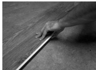
Fig. 4 – Angle long side into prior row.
