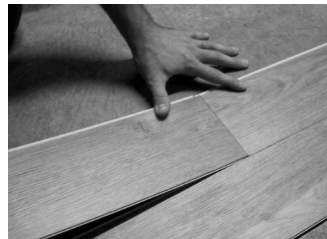
Fig. 5 – Angle end of next plank.
