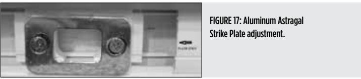
FIGURE 17: Aluminum Astragal Strike Plate adjustment.
