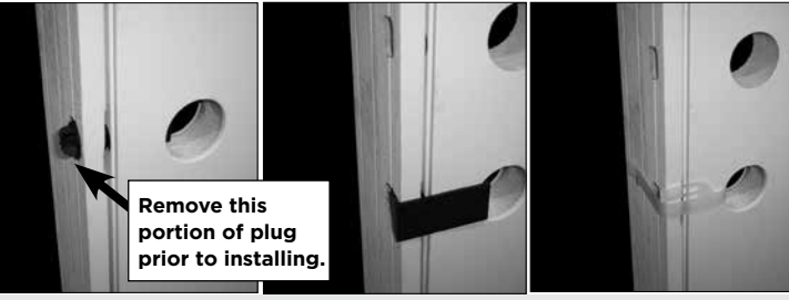
FIGURE 4: Some door units may be supplied with a "clip" or "plug" holding the panel aligned and closed during the initial installation steps. Do not remove at this time. Some door units may be supplied with a double headed nail or screw holding panel closed - this needs to be removed at this time.
