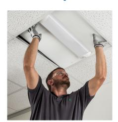
With its low-profile design, the BLT troffer offers greater installation flexibility, especially in applications where plenum space is limited.
