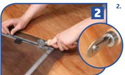
2. Using concave end of screen tool, insert spline at one corner and roll into groove over screening. Place hand on screen surface to hold screen straight. Roll spline into groove on all four sides.
