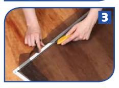
3. Trim off excess screening with utility knife on outside edge of the spline groove.
