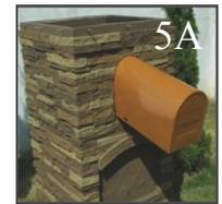
B) Drive 4 -2" screws through the top of the mailbox mounting plate (3rd bracket) into the top of the post. Slide the metal mailbox back over the mounting plate. Align the holes in the mailbox with the preset threads in the mounting plate.
