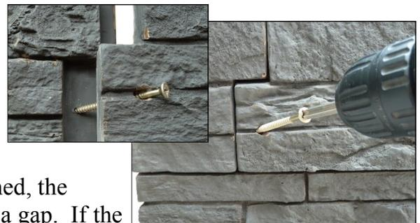
**Note to Installer:** Do not over tighten the screws when attaching the corner pieces. When over tightened, the corner piece will “kick out” at the bottom and create a gap. If the gap is present, pull the corners together to minimize the gap, then face screw through the female tongue, through the male base plate, and into the substrate. Use a 3" deck screw for this purpose. Use NextStone™ caulk to fill screw head and NextStone™ touch up paint for a professional finish.
