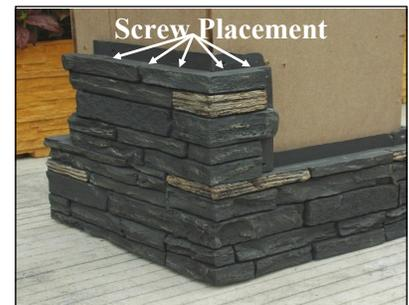
**4) Attaching the Corners-** There are 3 screw points on the long side of the corner, and 2 on the shorter end. Make sure to use 5 screws per corner. Hold the bottom edge of corner snug against the substrate while placing the screws to prevent over tightening of the screw hem. This prevents the bottom edge from kicking out.
