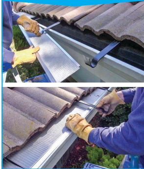
VILA TILE ROOF
