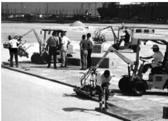
Figure 9. Mechanical installation equipment places concrete pavers rapidly.
