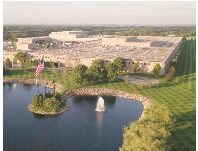
CAMBRIA PROCESSING FACILITY Le Sueur, Minnesota
