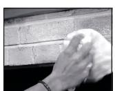
subsequent sections of bricks until the entire surface is covered. **Note:** The wiping step will allow some of the brick's original colors to come through. As the paint dries, the natural colors of the bricks will start to show through your application.
