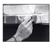
Using the provided 2" Brush, brush on your whitewash mixture starting at the top and working your way down. Only apply the paint to 4 to 6 bricks at a time. Once applied in that section, use the provided Wiping Rags to quickly wipe off the painted area.
