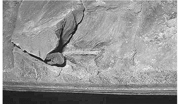
Counter Rotating Damage
