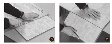
**Cut Palisade tiles** by scoring and snapping with a utility knife (image 6, 7). This method may require sanding the snapped edges.
