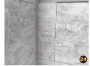
Use a damp rag or paper towel to clean off any sealant or adhesive that may have been squeezed onto the tile surface.
