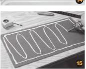
Apply the panel to the substrate by pressing it into place. Apply even pressure with your hands across the entire panel. If necessary, use painter's tape, shims or pins to hold panels in place until adhesive sets.
