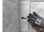
Apply sealant to the interlocking edges if this installation is for a wet environment.
