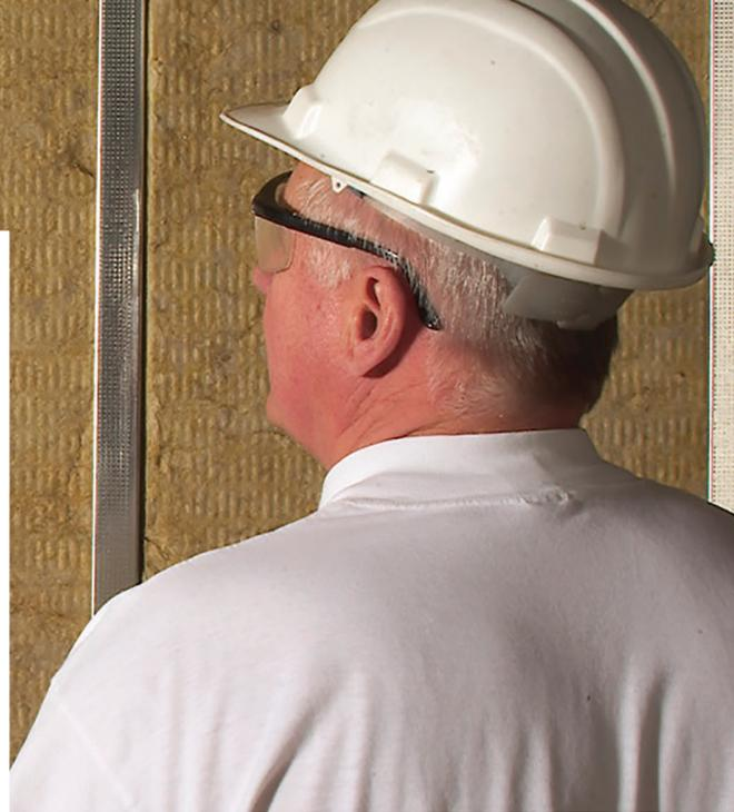
Thermafiber® Fire & Sound Guard® Plus is a hybrid light-density mineral wool batt that is designed to use in both interior and exterior wall cavities. This product combines the attributes of Thermafiber® UltraBatt™ and Thermafiber® Fire & Sound Guard® into one product, saving time for the installer.
