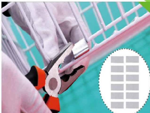
Secure with metal sheets
