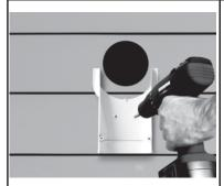
1. Determine the path which the lineset will follow and strike a chalk line to mark the surface material. Attach the base of the wall inlet, along the marked path. Predrill contraction. Install and where necessary. Duct must terminate with a sliding out of position.
