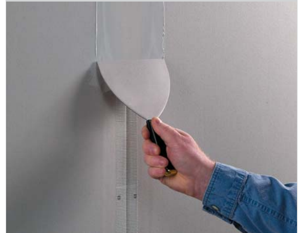
Self-adhesive tape saves time by eliminating the need for a pre-bedding coat.
