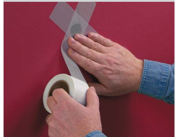
Self-adhesive tape saves time by eliminating the need for a pre-bedding coat.
