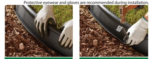
Place the edging into the trench, so that the bead on top sits at ground level. The lip can face either direction. Assure the straight side of the wall sits firmly against the dirt.
