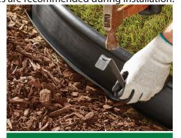
Hammer steel anchoring stakes at a 45° angle through the edging wall no more than 5 feet apart. Pack dirt into the lip and firmly against the edging wall. Backfill with desired ground cover.
