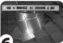
Rotate top of elbow to level position
