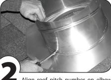
Align roof pitch number on elbow Place 3 screws through holes that line up tapping roof. with predrilled holes in base.
