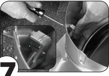
Place locking clamp across seam and tighten as shown with included screw.
