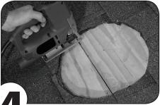
Cut hole as marked. Seal around
