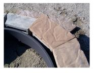
**Step 5**: Install the caps (8 units). Place the first top cap directly over one of the blocks in the second course allowing the cap to overhang the front of the block by about 1.5". Continue around the circle making slight adjustments as needed so that the edges of the caps fit tightly in the circle. Once the caps are in place remove them one by one and glue as above. Install clean porous rock or gravel between the steel ring and the blocks.
