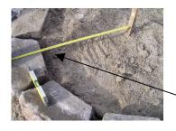
**Step 2**: Install first row of block (8 units). Using a center stake, lay out the blocks in a 16" radius from the center stake to the center of the back of each block. Level the blocks from front to back and side to side. Blocks may need to be shifted slightly in order to get a tight fit between all the blocks on the first course.
