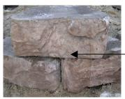
**Step 3**: Install second row of blocks (8 units). Place the first block on top of the bottom block staggering the intersection of two blocks on the row below. Continue around the circle making slight adjustments as needed so that the edge of the blocks fit tightly in the circle.
