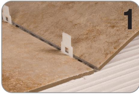
Slide two clips under the tile and into the mortar approximately 2" from each end of the tile. Place the second tile.
