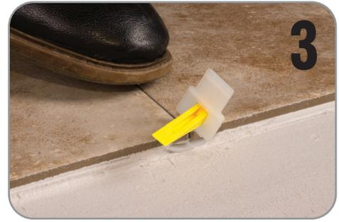
Once mortar has set, simply kick the clips to snap off at the specially designated break-points. Save wedges for future use.
