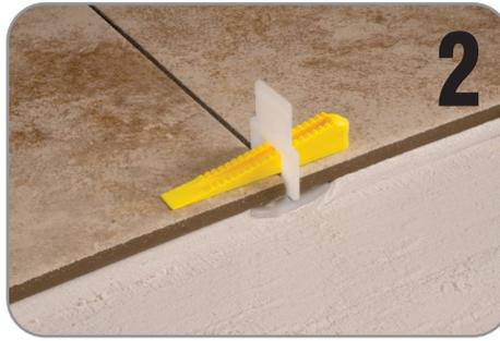
Slide the reusable wedges into the clips to **LEVEL, ALIGN, SPACE** and **HOLD** the tiles.
