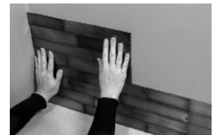
When placing tiles on the second row and beyond, angle the tile back about 30 degrees and rest the bottom edge on the tile below, then slide it over to abutt the previous tile.
