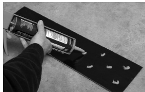
Method 2 - Using high-quality polyurethane construction adhesive
