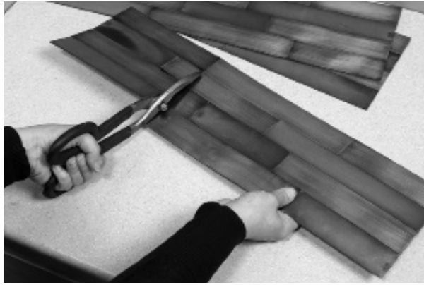
Cutting a straight cut with a snips
