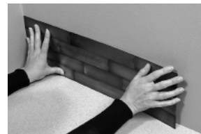
Place the first tile. Angle side or top of tile away from wall until you are sure of placement. Use the counter top as a guide as you move it into place.
