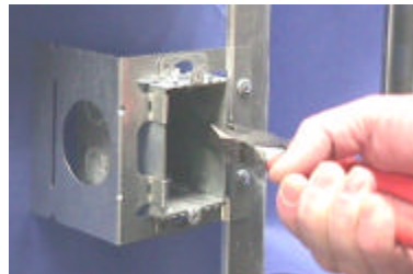
CRIMP TABS TIGHTLY ON BOX
