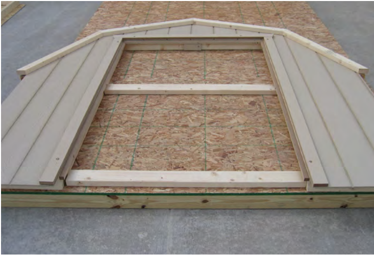
54. Make sure the rakes are all installed and fastened with 3" nails.
