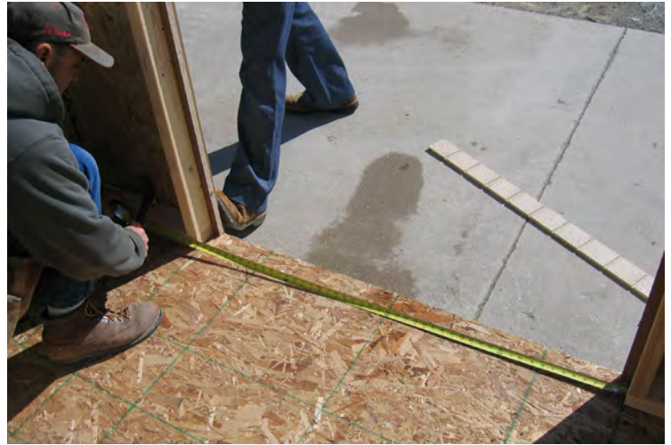
73. Make sure you have 48" or 60" (depending on building width) in between the door opening, 48" on 8' wide buildings and 60" on 10' and wider buildings.
