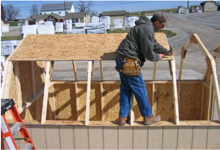
84. Secure with 2" nails as shown.
