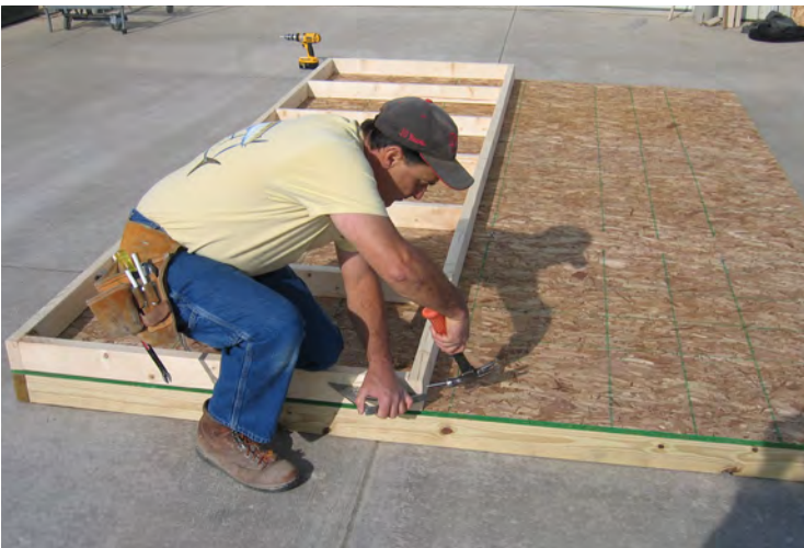
15. Build the next wall as shown.
