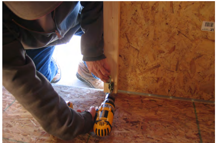
95. Install the barrel bolt, using 1 1/4" screws, on the inside of the left hand door (facing).
