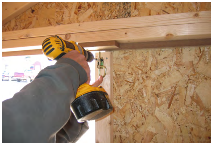
96. Then install the barrel bolt at the top of the door.
