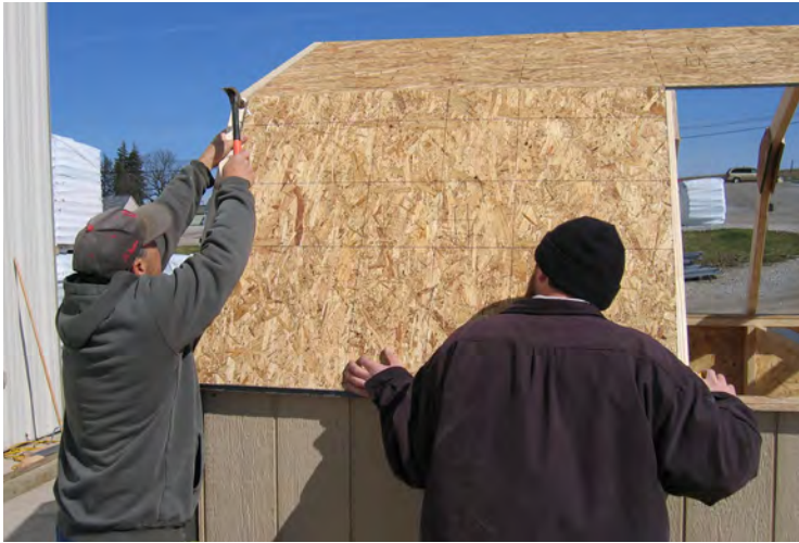
90. Continue with sheathing.
