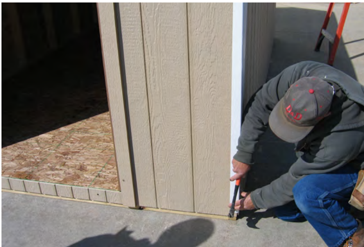
92. Next install aluminum corners and secure with 2" nails.
