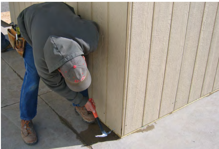
70. Fasten the bottom with 2" nails every 8 inches.
