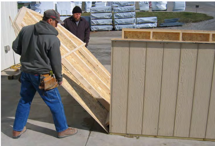
68. Next install gable wall.
