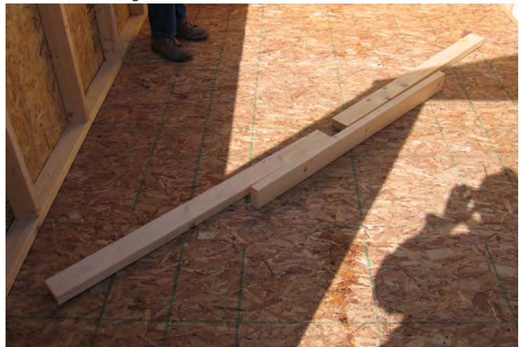
75. Locate the temporary wall braces.
