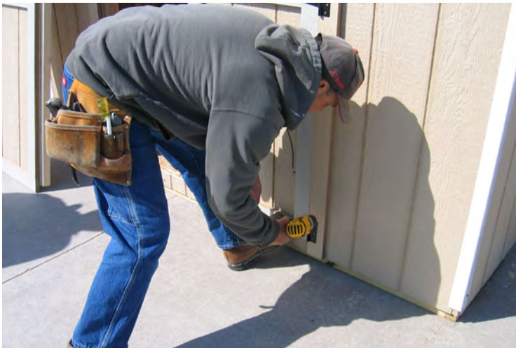
94. Fasten the hinges on the top, middle and bottom.
