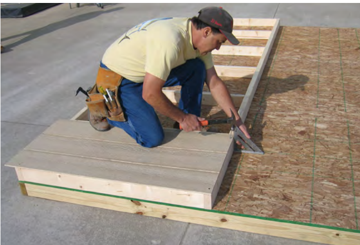
17. Make sure that you always fasten the top first and keep flush with the 2x4 top plate.
