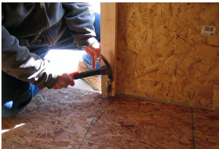
97. Use your hammer to tap on the barrel bolt to locate the mark.
