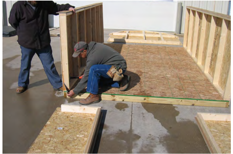
67. Continue with walls.
