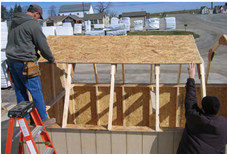
82. Install the first piece of sheathing as shown.
