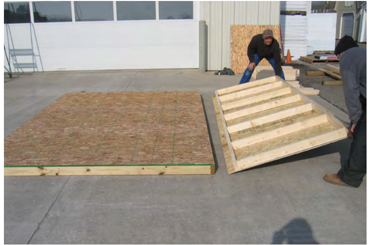
14. Lay wall off to the side as shown.
