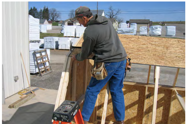
83. Secure the outside corner with 2" nails.
