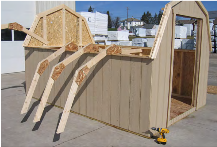
78. Hang trusses on the walls.
