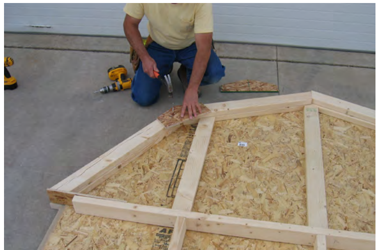
59. Install OSB gussets, as shown, and secure with 2" nails to start truss assembly.
