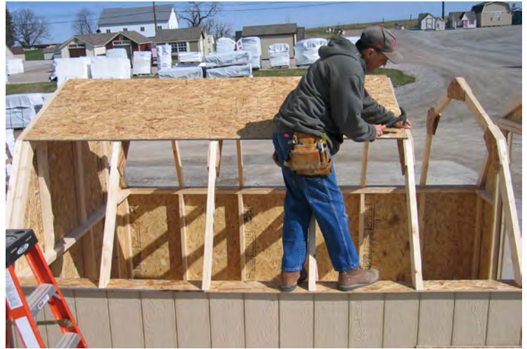
85. Make sure the trusses are 24" on center before fastening.
