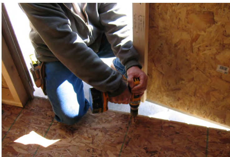
99. Now use your 5/16" drill bit to drill the hole.
