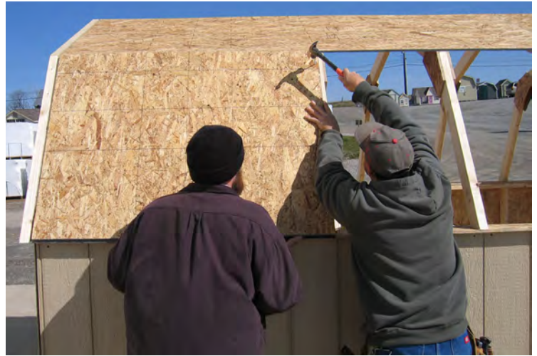
91. Continue with the sheathing.
