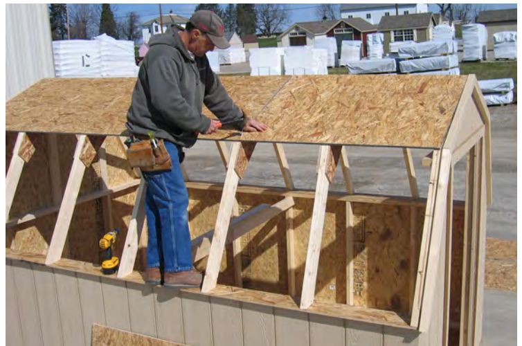
87. Continue with OSB Sheeting and fasten every 6" to 8" with 2" nails.
