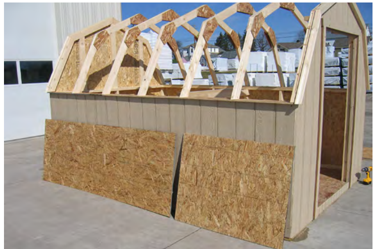
81. Locate OSB sheathing for the roofing.
