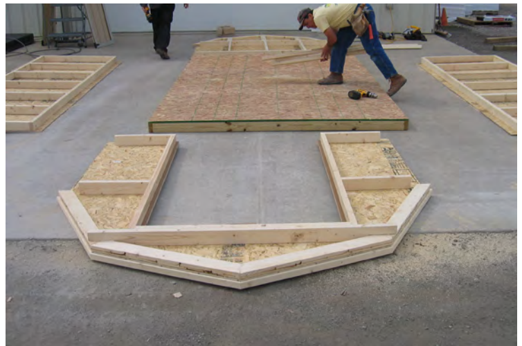
57. Lay wall off to the side.
