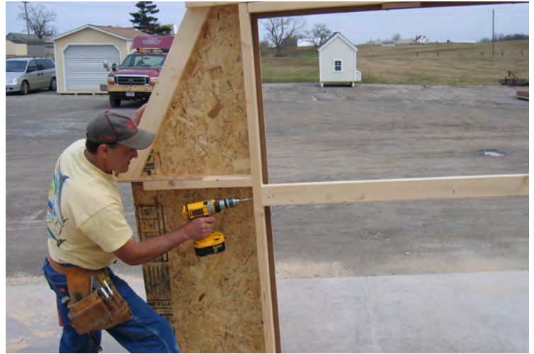
55. Remove 2x4 brace. Top and bottom.
