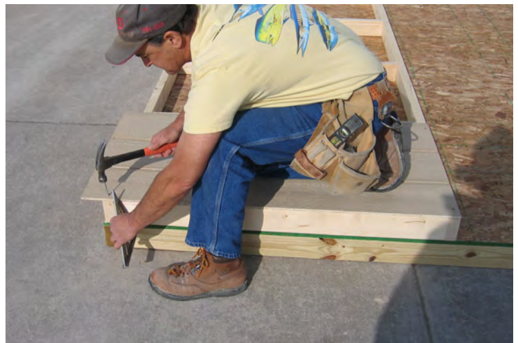
18. Continue installing the Smartside siding.
