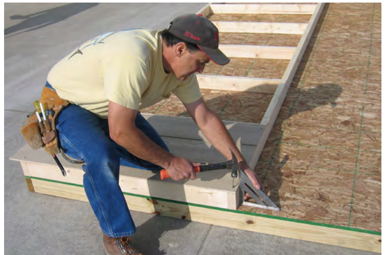
16. Continue installing Smartside siding, making sure all is flush.
