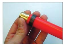
2. Slide crimp ring over end of tubing. Insert fitting into end of tubing until it stops. Position the crimp ring 1/8" to 1/4" from the end of the tubing and over the ribs of the fitting.
