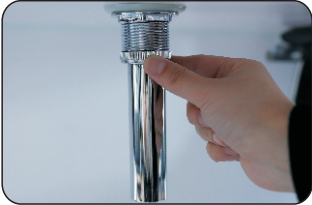
Contact two parts of the drain and tighten
