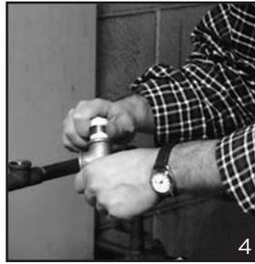
Point the opening on the side of the tee to the front or to the side so that it is easily accessible. (Fig. 5)
