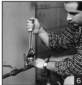
8. Attach a pipe or hose to steer any emergency overflow water away from the electrical connections of the pump if necessary. **Do not install a plug or valve or insert anything else in the pressure relief valve that would obstruct the flow of water from it. This can create a serious safety hazard in your home.**
