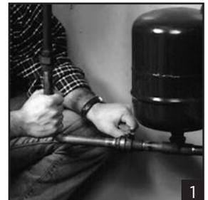
3. Close the ball or gate valve on the supply line, the pipe which supplies water to the plumbing inside your house. (Fig. 1) This stops water running into or out of the plumbing in your house.
