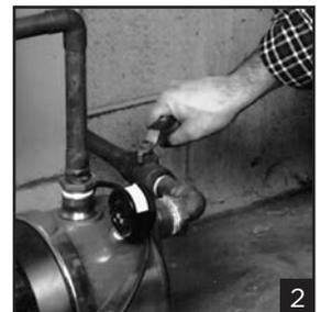
4. Close the ball or gate valve on the pump feed line, the pipe through which the pump draws water from the well into the house. This stops water from running back into the well. (Fig. 2)
