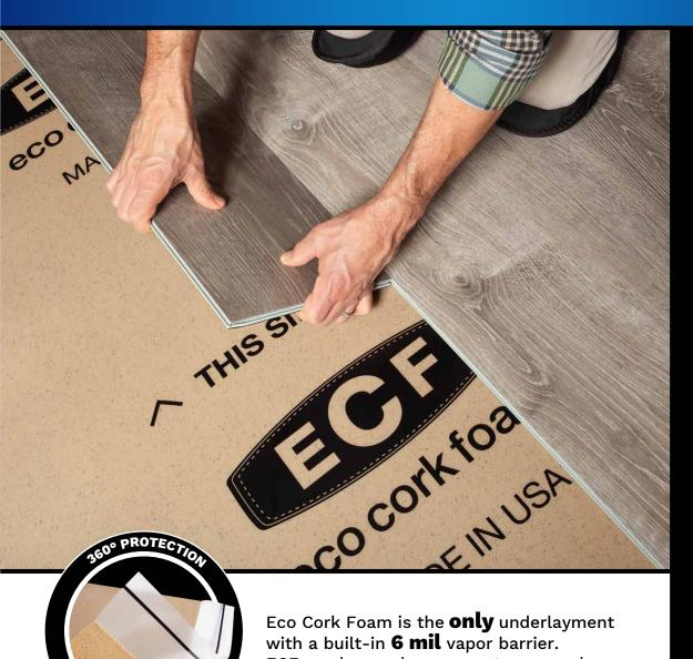
Eco Cork Foam is the **only** underlayment with a built-in 6 mil vapor barrier. ECF can be used on concrete or wood subfloors on any level of your home.
