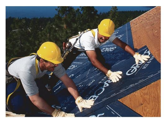
GRACE ICE & WATER SHIELD® fully-adhered smooth surface roofing underlayment provides best in class roof leak protection. Its proprietary and time tested rubberized asphalt formulation has been proven to form a watertight bond with the roof deck and to seal around fasteners used to attach roof coverings. When it comes to roof protection, insist on the original – GRACE ICE & WATER SHIELD® roofing underlayment.
