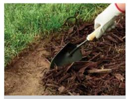
Clear the installation area of all grass, loose soil, mulch, and other debris. Place aluminum edging on the cleared installation surface with the anchoring tabs facing the planting bed.
