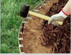
Use a rubber mallet to pound anchoring spikes (included in kit) through the aluminum tabs to secure the edging. If needed, additional anchoring spikes are sold seperately.
