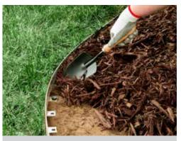
Backfill to the top of the edging with mulch, river rock, wood chips, or other preferred ground cover.
