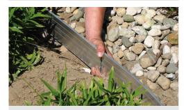
4 Slide ends of edging strips together to connect pieces. Adjacent section of edging can be connected prior to or after the sections are in place.
