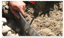
Drive spikes through holes in edging at a 45 degree angle.
