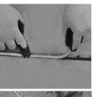
Take the cut **CRACK•STIX**<sup>®</sup> and push it down into the crack/joint inch by inch, until it is approximately 1/8" from the top of the surrounding concrete surface (slight recess for expansion & contraction). Light the propane torch & adjust the total flame until it is about 3-4" long & the bright blue tip of the flame is 1" long. Do not touch the flame, it is
