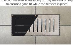
8. Adjust the height of the diffuser plate to allow the vent to lay perfectly flush and screw in place. (Full details are in the video link below.)
