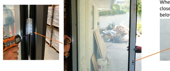
When the door is closed holes in picture below must be inside.
