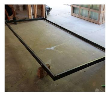
Once frame is assembled, place it by the installation location and check the opening size and Floor level
