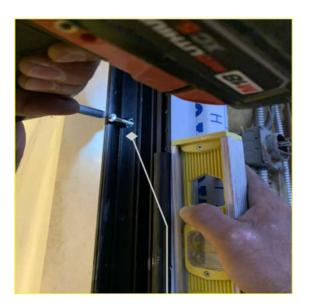
2. Drill 7/16 hole into first layer of Side frames for cap and ¼" hole on the other layers.
