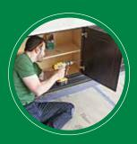
CONNECTING AND SECURING CABINETRY FROM KEN HARRIS @KH\_WOODWORKING
